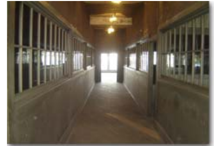
Harry Burt/Ross Radio Building Third Floor Hallway lined with windows for the public to watch the candy making process.
